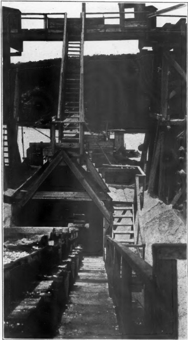
Belt Conveyor from Scalping Screens to Sizing Screens
